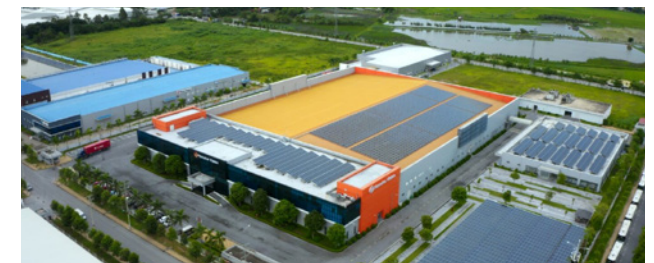
Solar panels at the Vietnamese subsidiary
