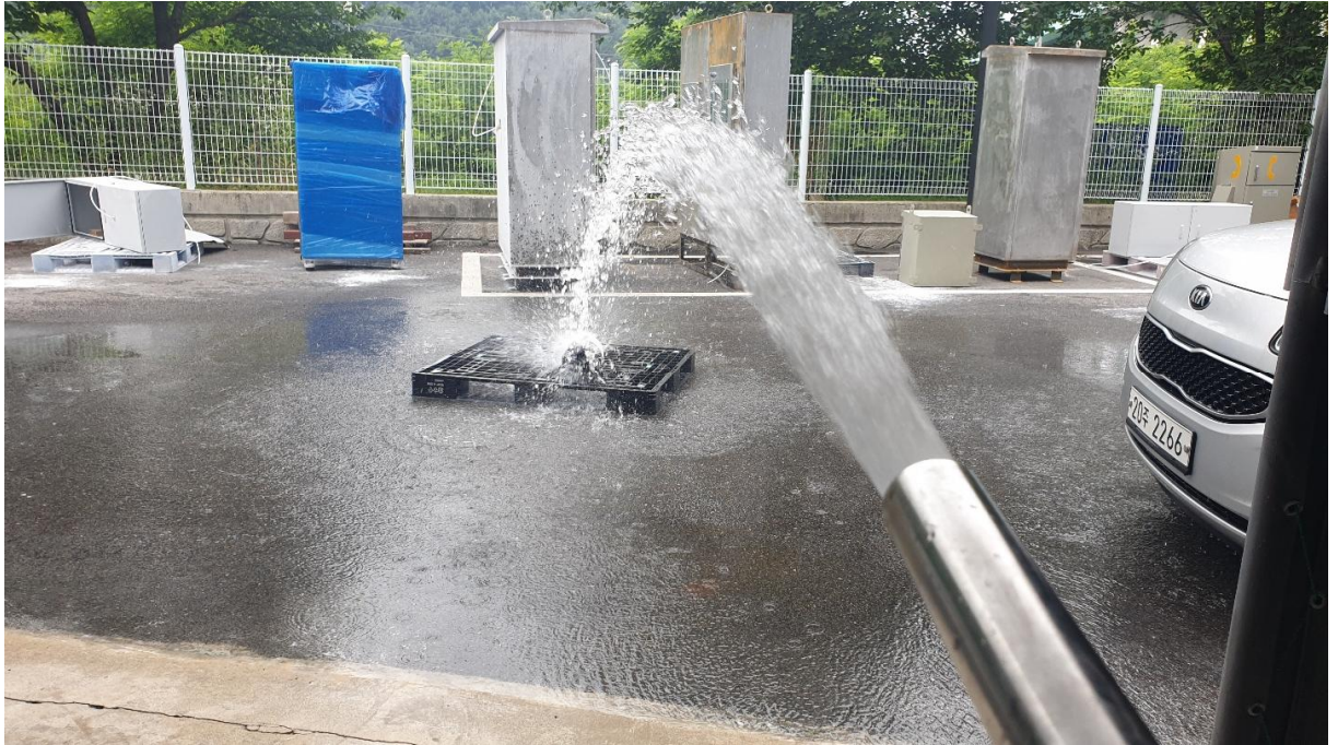
<Photo 3 > Hose down test
